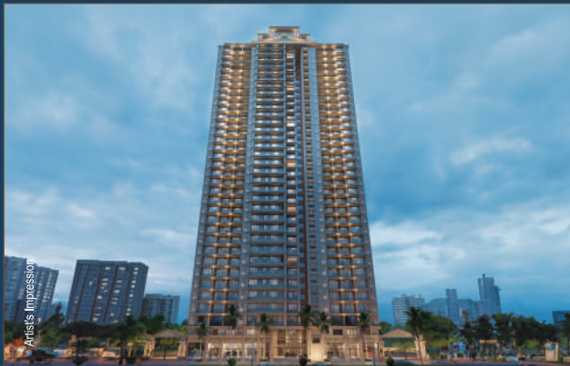
SAI PLATINUM KHARGHAR
